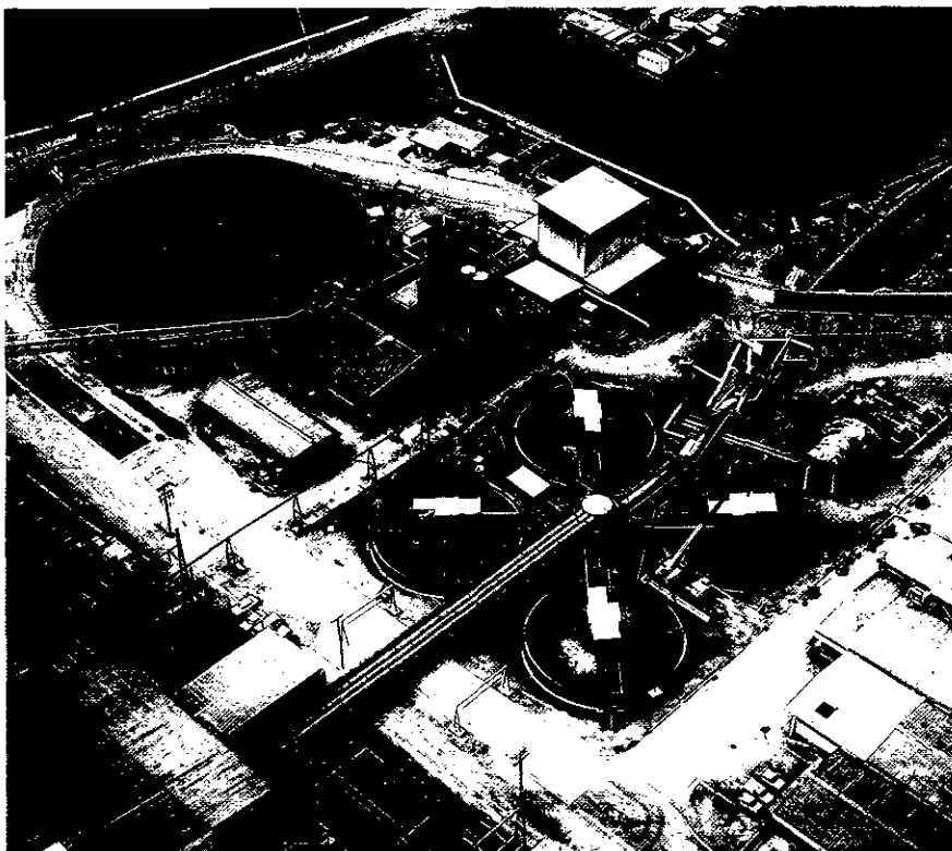
The new tailings water reclamation system uses four 24.5 metre diameter Enviro-Clear high capacity thickeners to recover water from the concentrator tailings slurry. The availability of reclaimed water has significantly reduced the power required to pump water to the concentrator and has eliminated water shortages.
